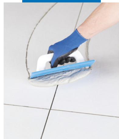
Spreading Ultracolor Plus on porcelain floor tiles with a rubber float
