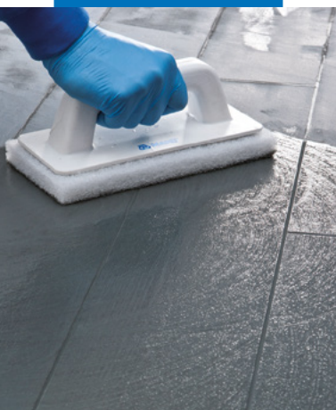
Cleaning the joints with a Scotch-Brite® pad (when the product is semi hardened)
