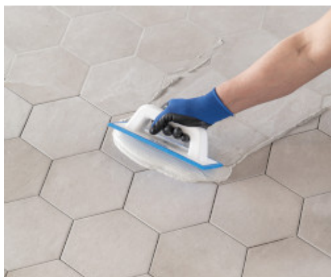
Application of Keracolor FF with MAPEI float
