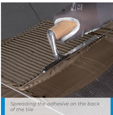
Spreading adhesive on the back of the tile
