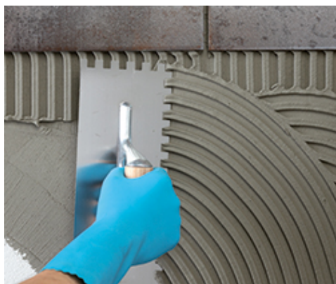
Spreading Ultralite S1 with a notched trowel on wall
