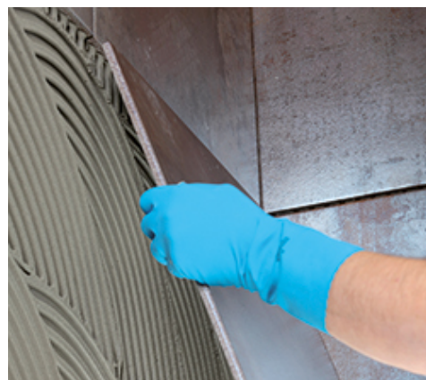
Laying large-sized tiles on walls
