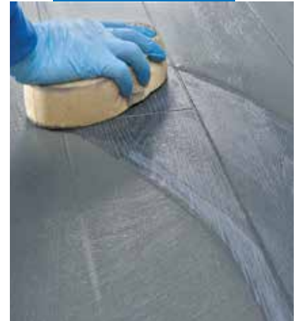
Cleaning and finishing the joints with a hard cellulose sponge
